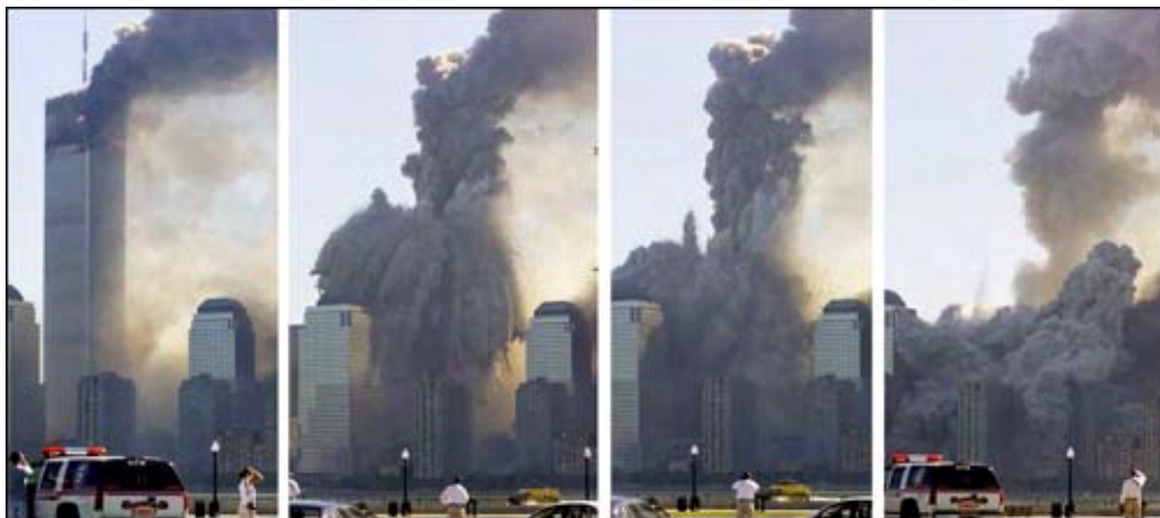
Fig. 10 Sequence of Collapse of North Tower ( Photo from CNN)
