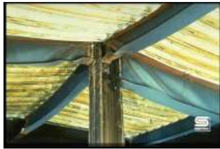
Figure 1. Flange-buckling and beam-web shear buckling in combination [3]
