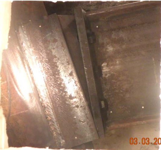
View of Camera 1
